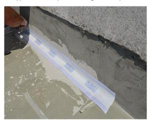
The AQUAZIP ONE waterproofing system will also be applied on the vertical overlaps, and after suitable curing will be covered with a coat of KI7 or KZ 35, lime and cement base coat plasters/renders for exteriors and interiors, mixed with a solution of water and AG 15 (1 part AG 15 to 3 parts water). The base coat plaster must be fine-float finished, embedding wide-weave synthetic plaster reinforcing mesh during application.
