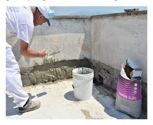
The AQUAZIP ELASTOBAND will be positioned along the connections between the horizontal plane and the vertical overlaps. The strip must be laid continuously on the application surfaces, first applying an at least 2 mm thick layer of AQUAZIP ONE waterproofing membrane, to a width exceeding the strip and making sure to leave the centre part free. For perfect sealing of the corners, use the appropriate preformed elements.
